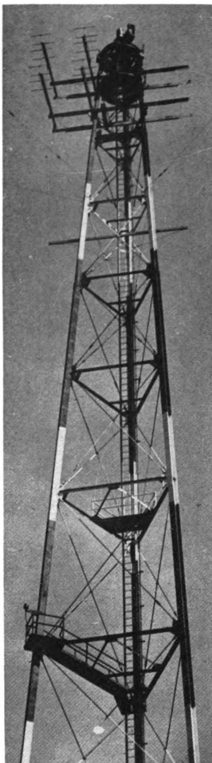
Radio link antennas under construction.
