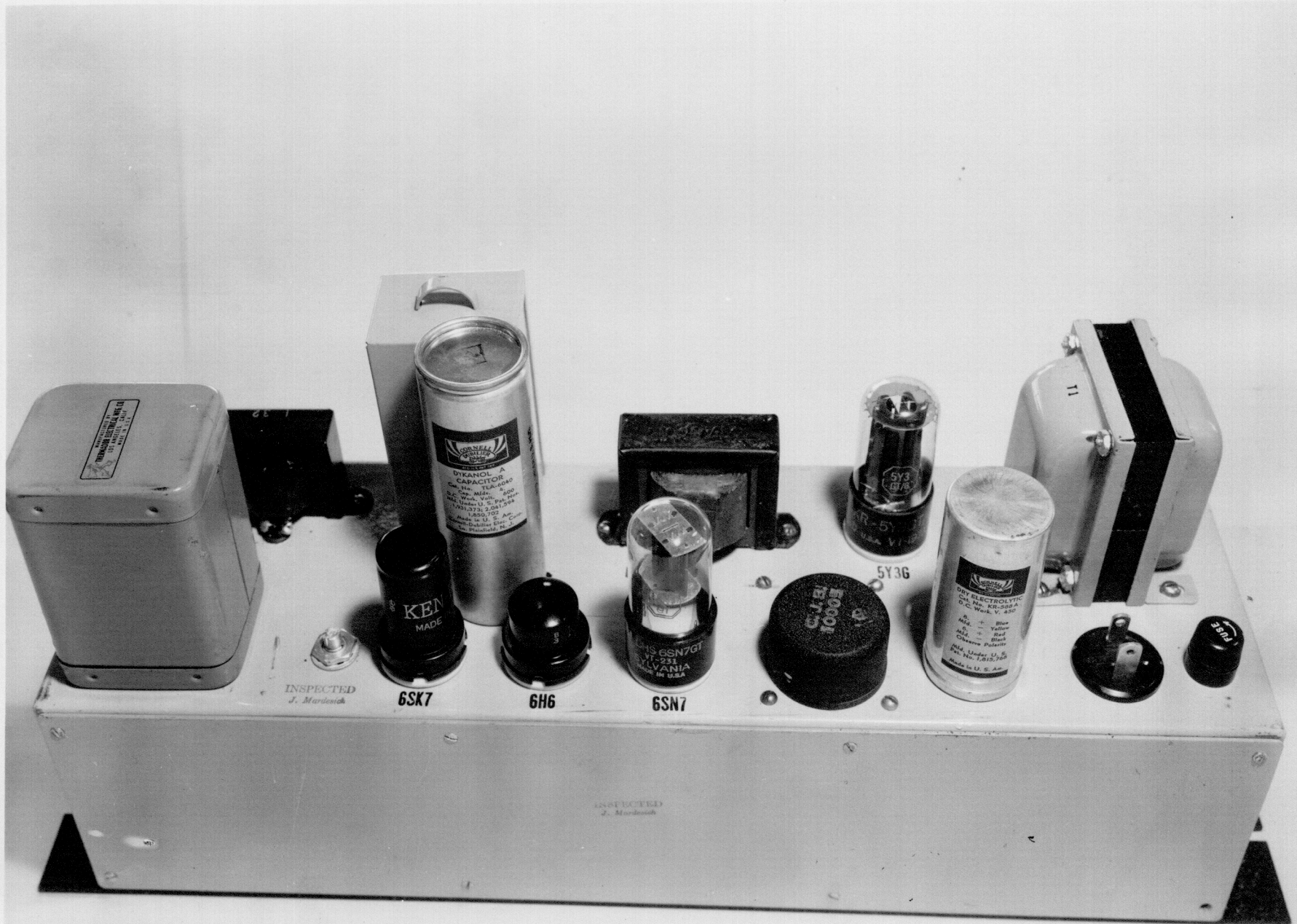
2507-45 Puget Sound Navy Yard 15 May 1945 Photograph (X) Localizer Monitor, Back View.
