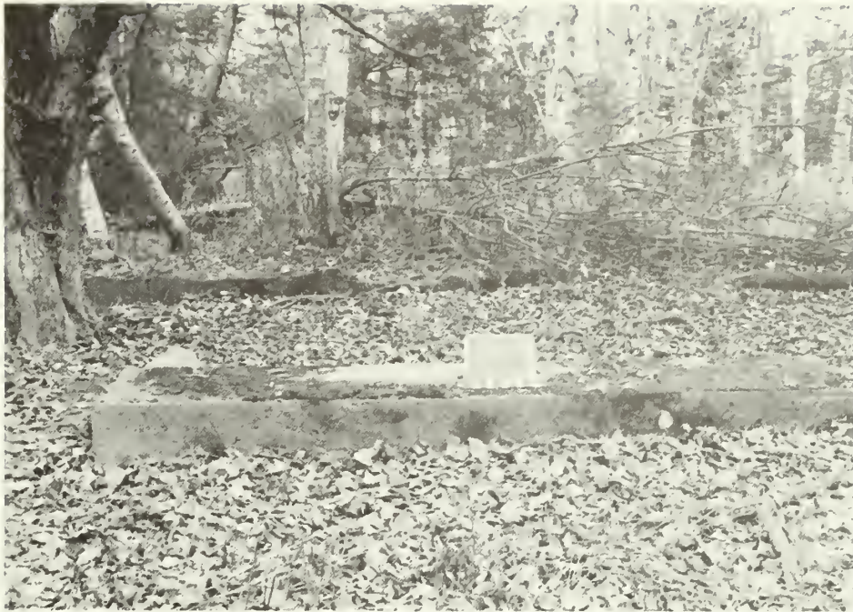
Photograph 41: Features 18 and 20, Barracks B steps and foundation
