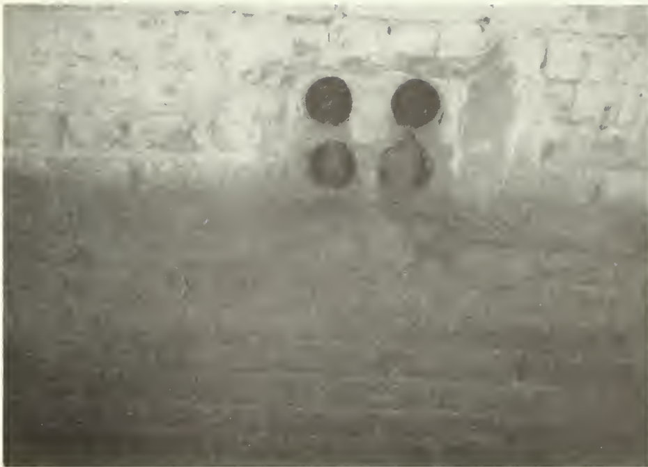
Photograph no. 61: Interior of Feature 7 showing electrical conduit
