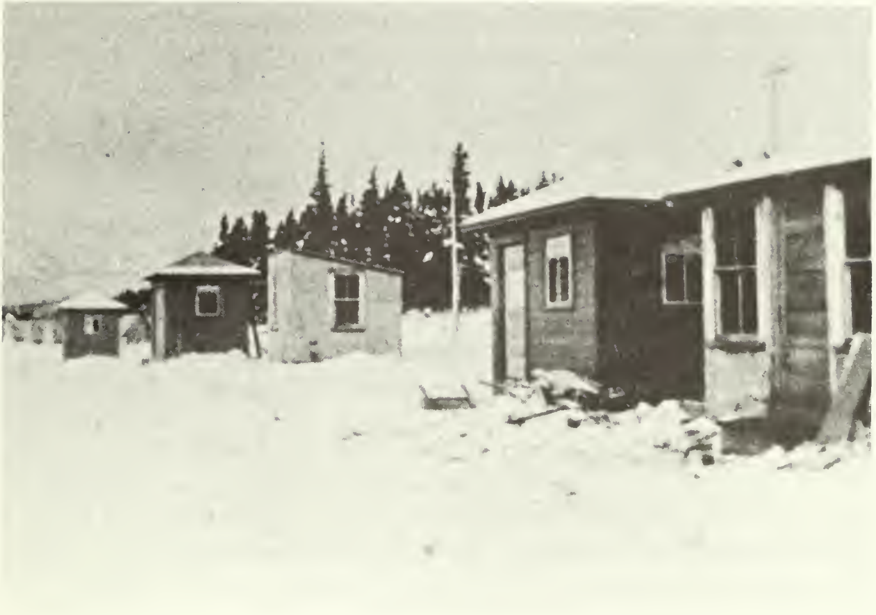
Photograph no. 17: Hoxie and receiving sheds
