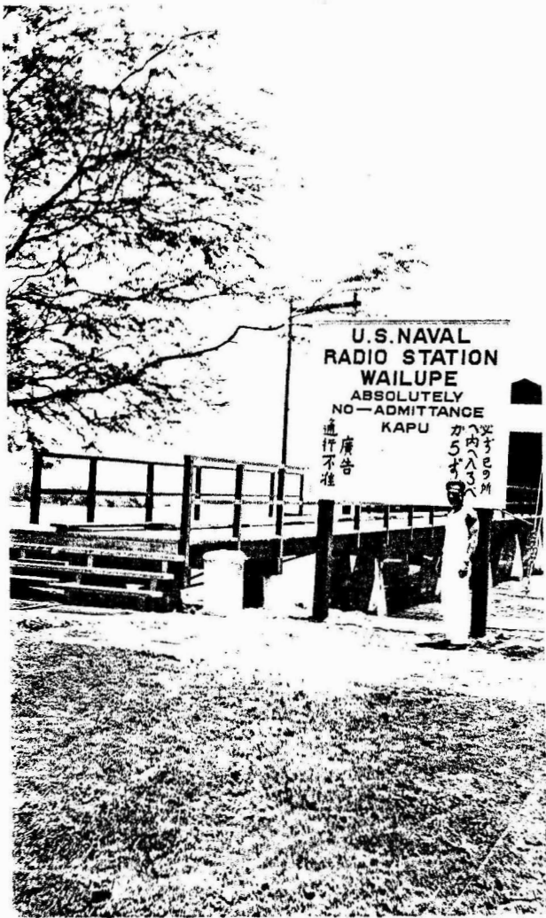
Bridge over the water, operating building C.R. "Shorty" Spicer, Wailupe, 1921
