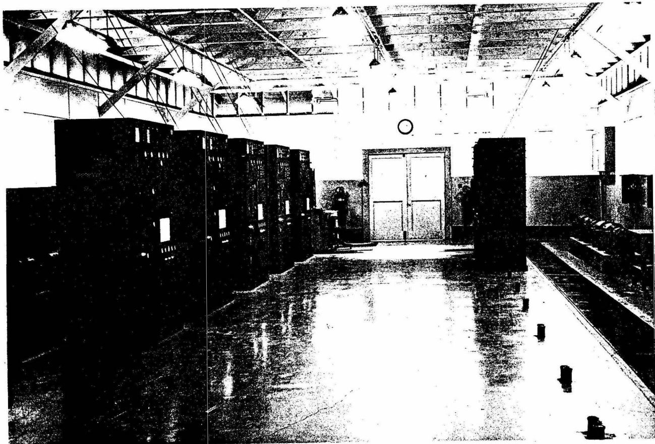
A few of the transmitters at Lualualei - NRM - 1944.
