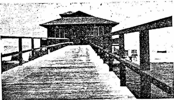
OPERATING BUILDING, WAILUPE
