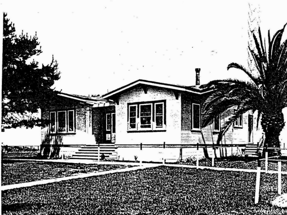
Navy Point Loma Radio Control Station 1927 1927
