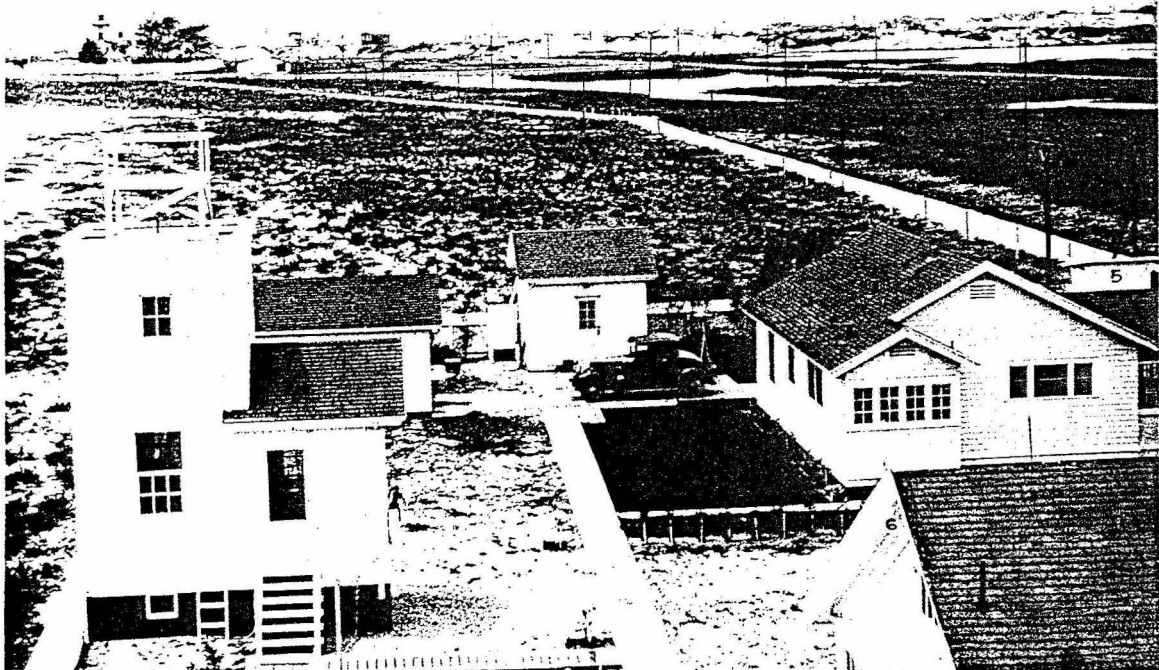
VIEW FROM TOP OF WATER TANK LOOKING WEST
