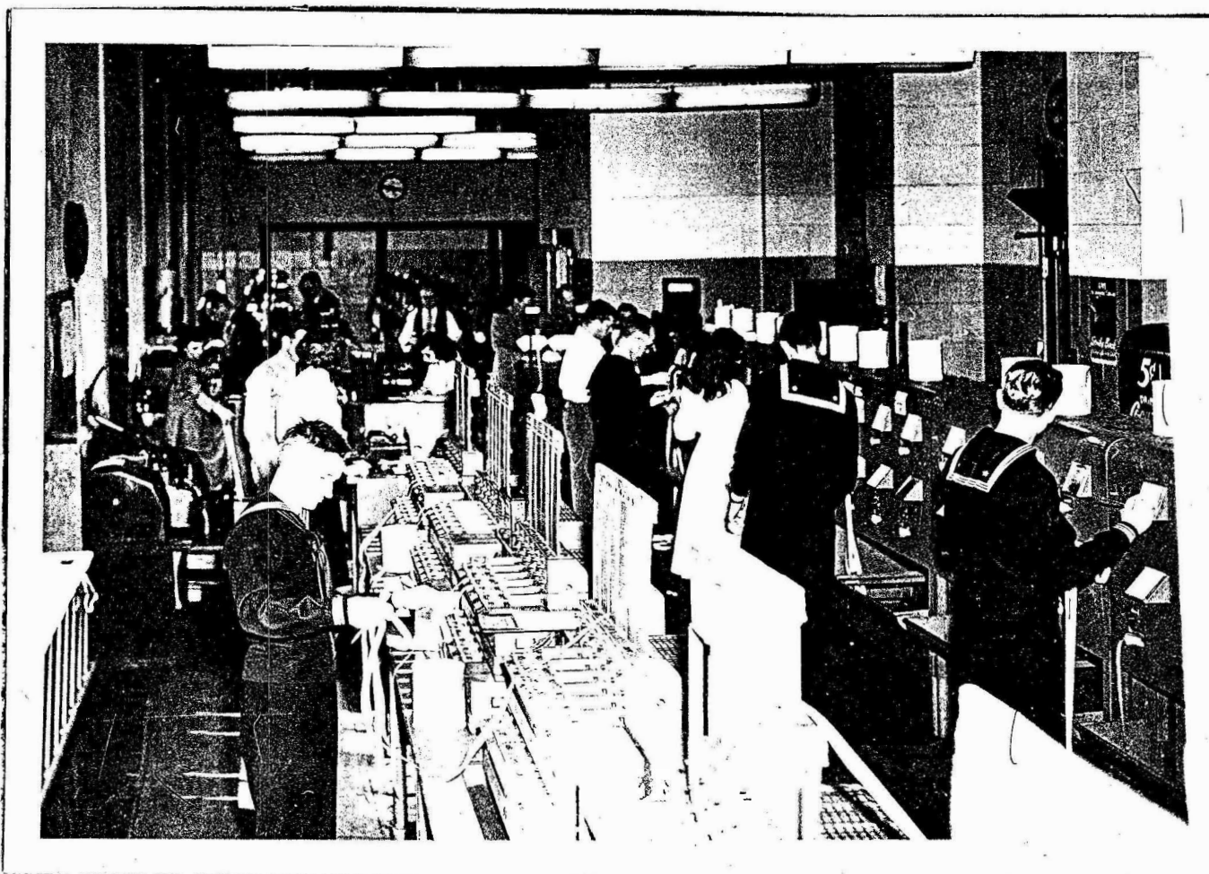
Teletype tape relay room, U. S. NAVCOMMSTA, San Francisco, California. Tape transmitters on left, receivers on right, tape record reels in back. 1952 Photo by Les Funston
