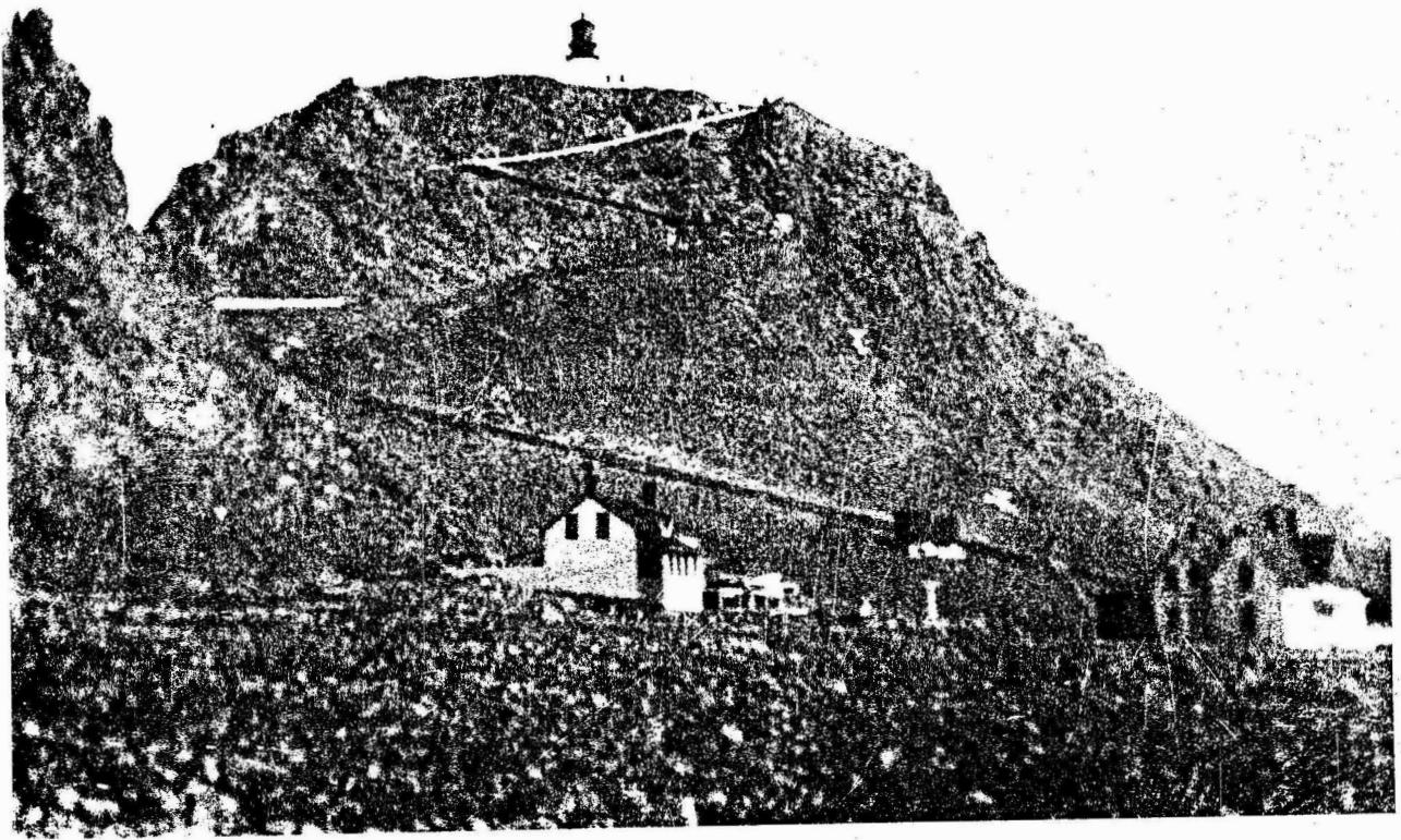
Lighthouse and tender's quarters. Note rails for hand-hold and guide in climbing to the light in dense fog at night.
