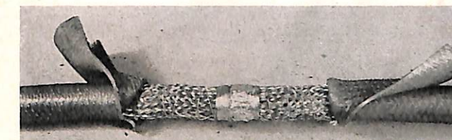
FIGURE 3—Cable prepared for splicing of jacket.
