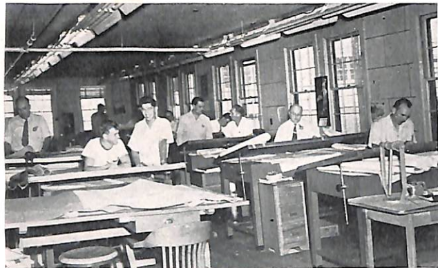
FIGURE 7—View of the Drafting Room.
