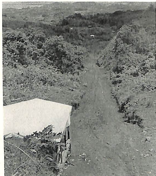
CLEARED AREA into which downleads are lowered. This area is in line with the center of the spans.
