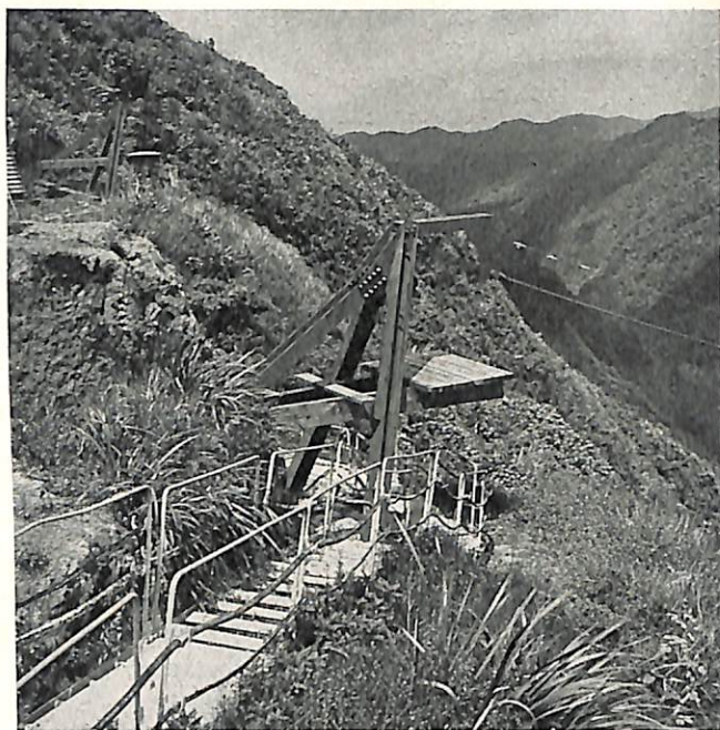
ANCHORAGES (Nos. 2 and 3), showing steel walkway which provides access to them.
