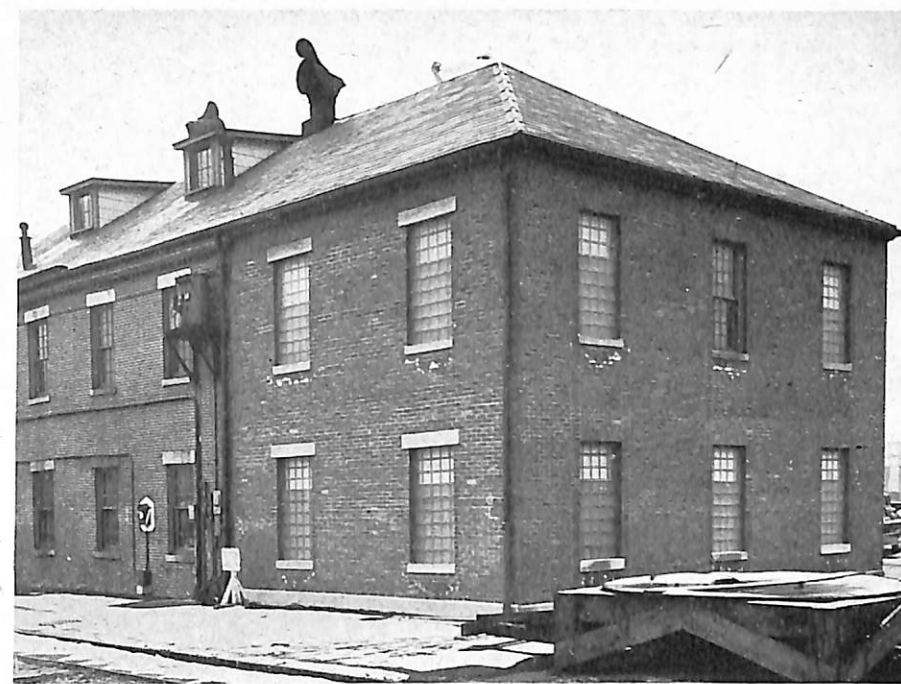
The Sonar Transducer Repair Facility. The test tank is housed in the right end of the building. This building has glass block windows.
