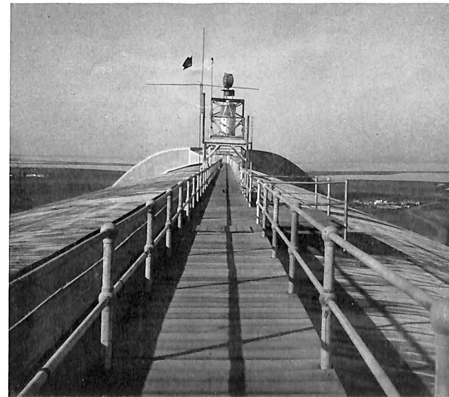
Check for the presence of metal fences in proximity to receiving antennas.
