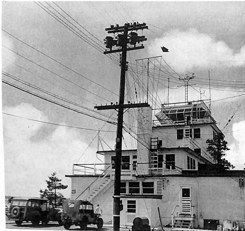
Check for power lines and transformers in proximity to antennas.
