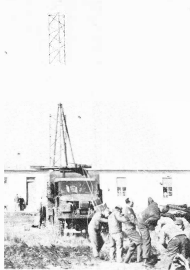
Antenna guy wires are set up by a NATO outside maintenance crew.
