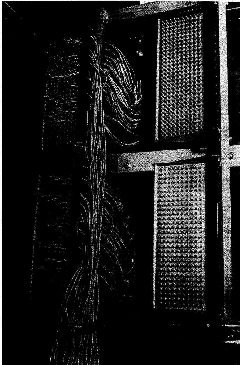
Figure 4-7.—Mainframe terminal boards.
