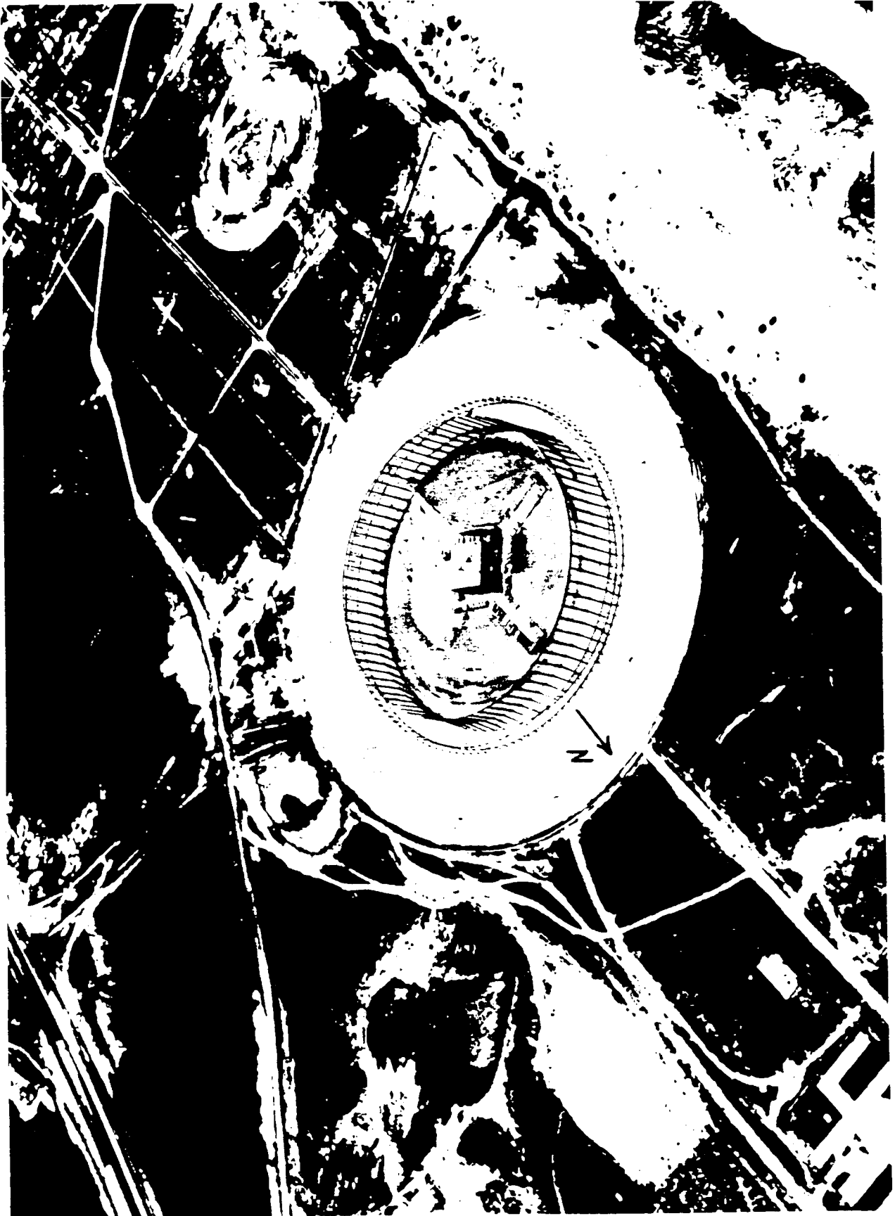
FIGURE 1-1. FRD-10 Circularly Disposed Antenna Array (Wullenweb r).
