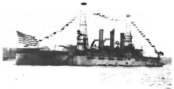
EARLY RADIO COMMUNICATION INSTALLATION— BATTLESHIP USS NEW JERSEY (1914)
