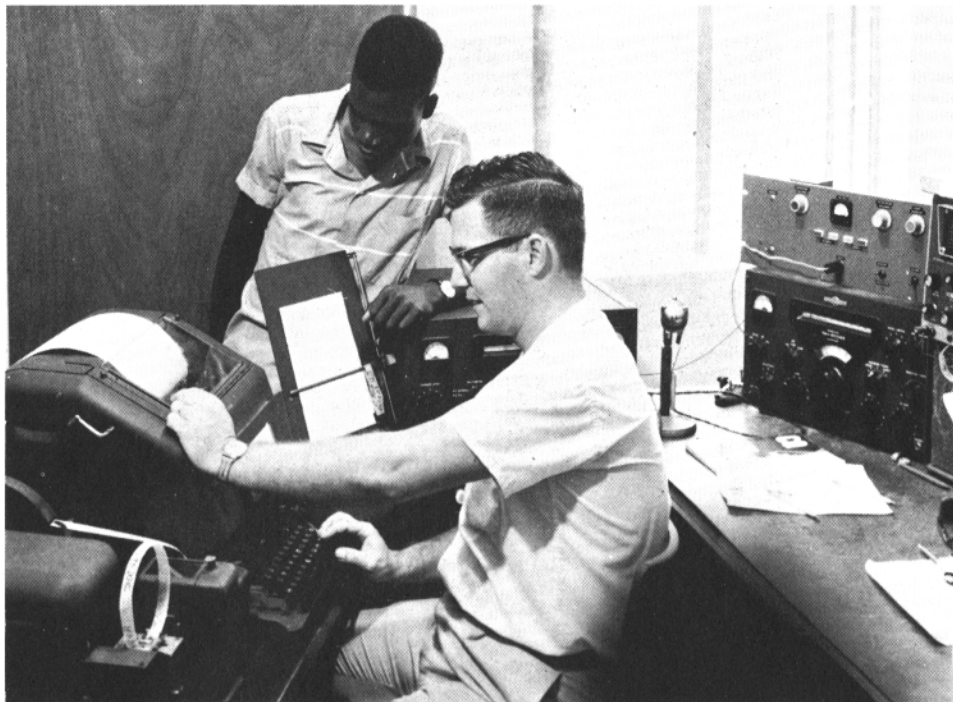
OBRA BLISS, EL2F MONROVIA, LIBERIA
