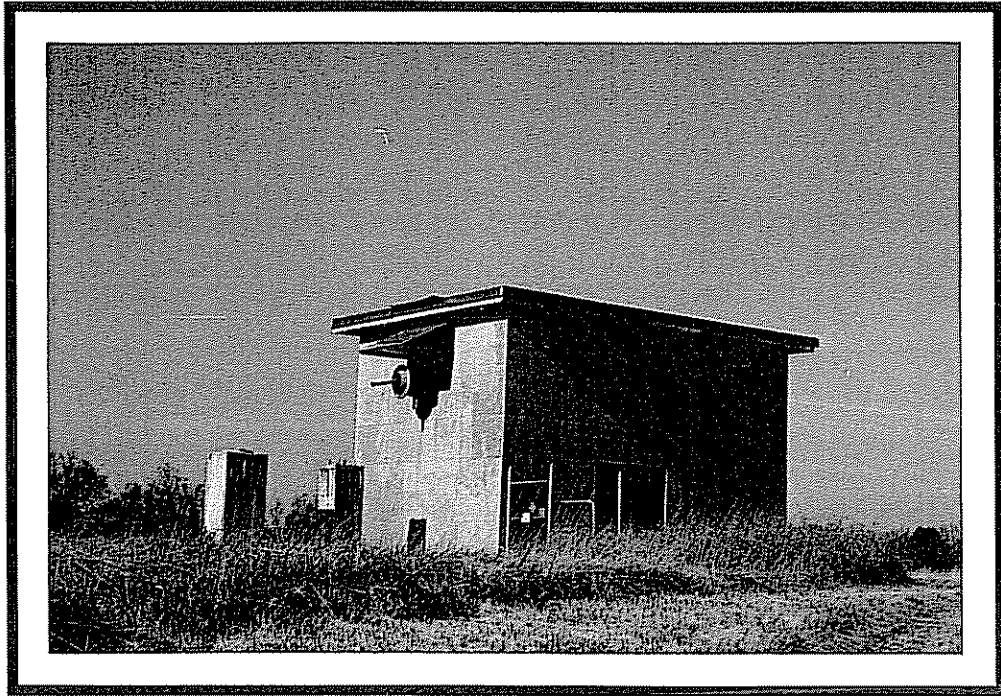
Figure 18. View of a typical 1950s helix house. Building D-11 was constructed at NRTF Driver to support an 800-foot vertical radiator tower.
